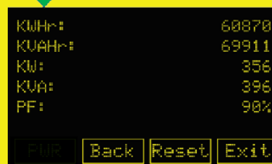
Power Metering Screen
