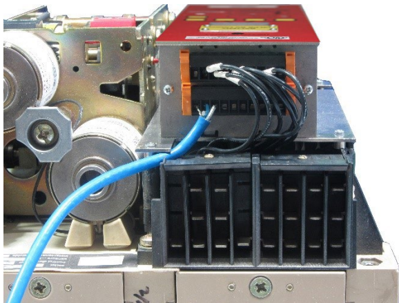
Communications Cable Installation (with cover removed) (AC-PRO-MP-II)
