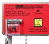
QT2-Switch on front of cubicle door
